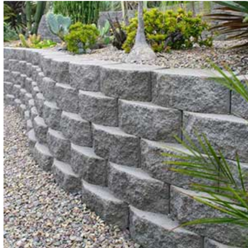
Landscape block retaining wall
