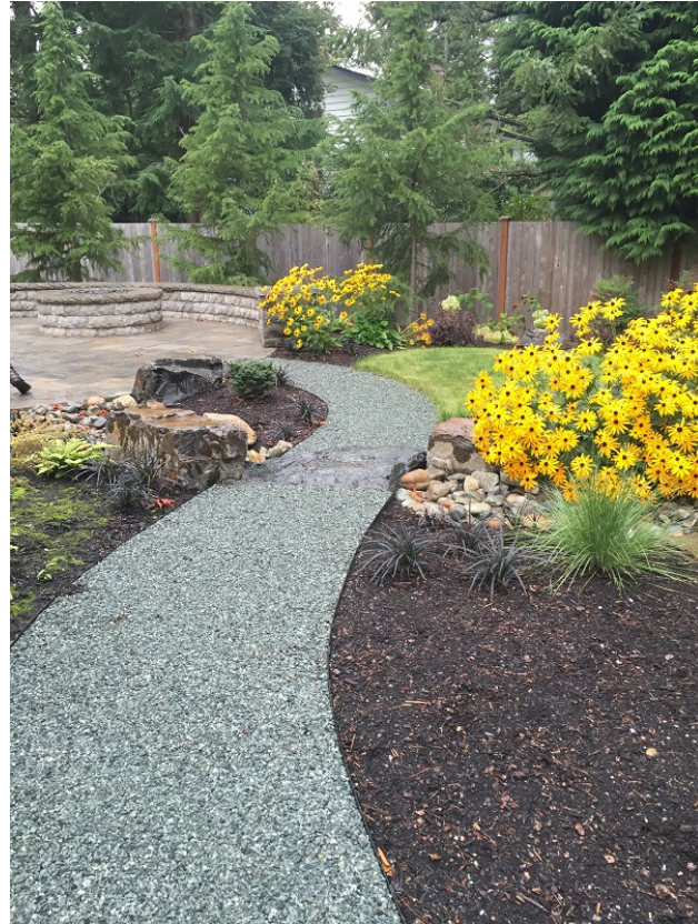
1/4 minus gravel pathway (with steel edging)
